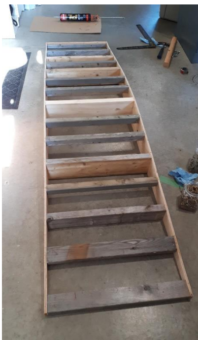
Figure 8. In-fill joists approximately every 6 inches.
