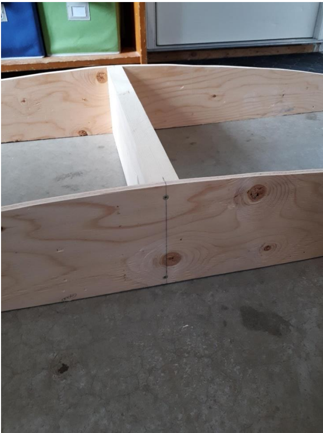
Figure 5. Placement of the central joist
