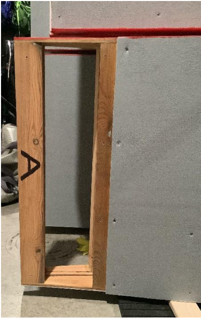
Figure 9. End section placement of decking
